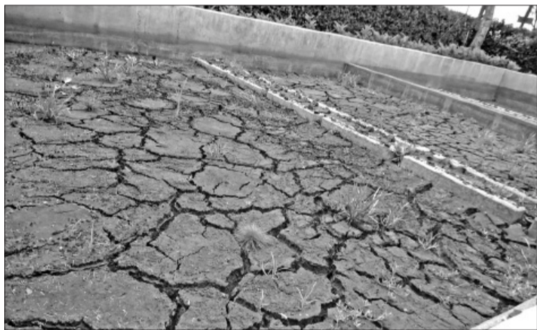
Sludge drying bed at Nyewasco water treatment plant at Kamakwa at the outskirts of Nyeri town. Photo/Joseph Mukubwa
