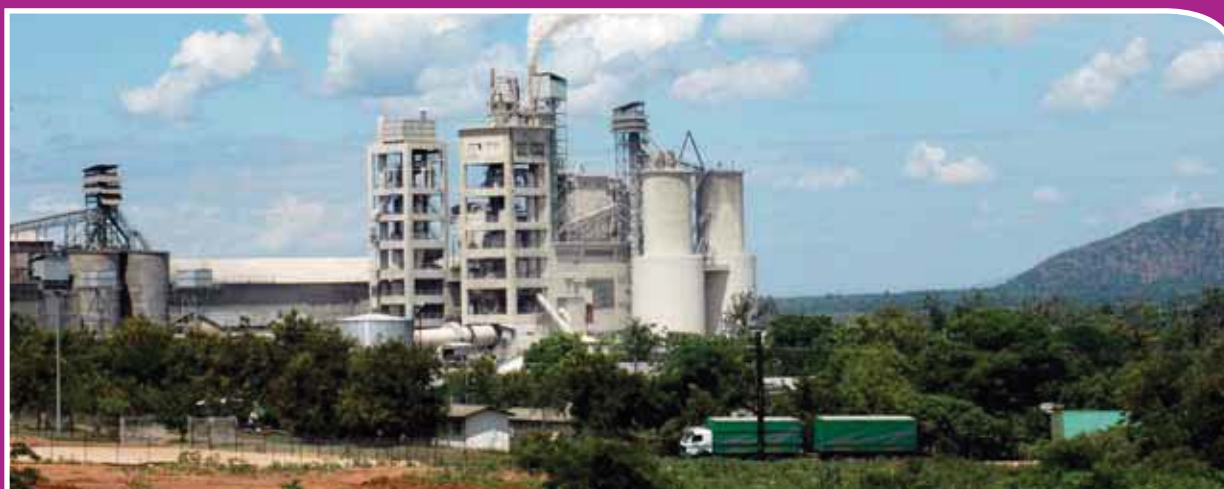
Cement factory in Hima
