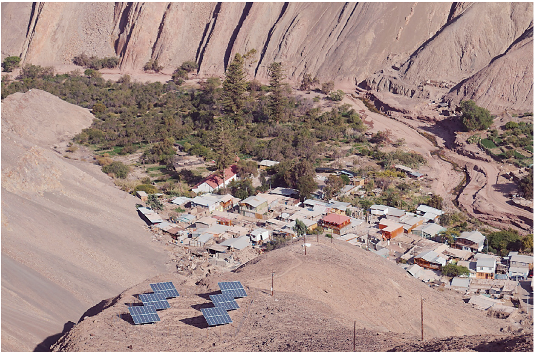
Chart nº 9: Solar panel installations that are part of the micro-grid in the community of Huatacondo.
