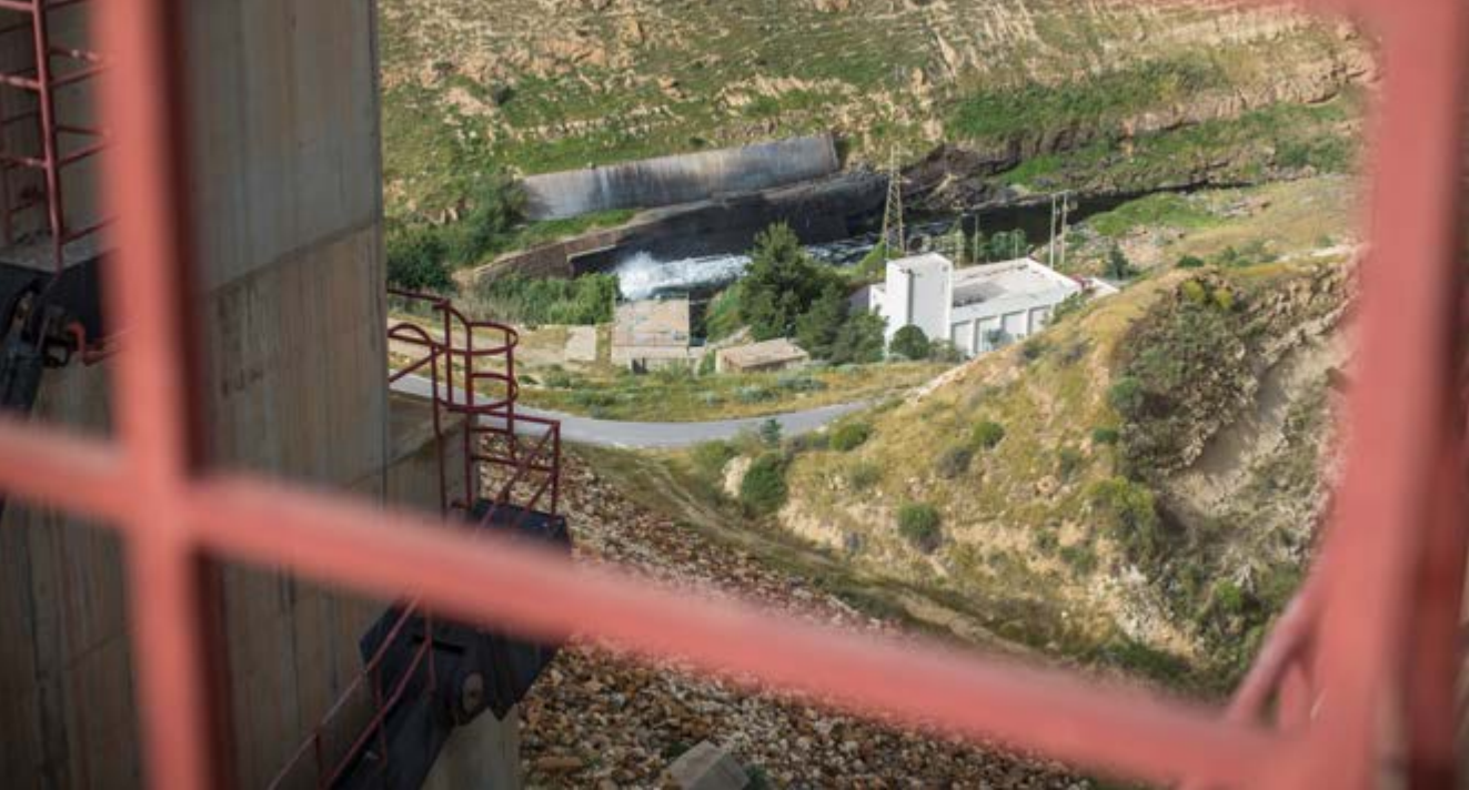
Water scarcity: The expansion of Jordan's water infrastructure is a focus of German development cooperation with the Kingdom. However, due to technical defects and theft, only half of the water produced reaches the end consumers. The picture shows a waterworks located at the King Talal Dam. Photo: © Thomas Imo, photothek, picture alliance.
