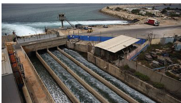
Figure 11: Brine water flowing into the Mediterranean Sea, passing through a desalination plant in the coastal city of Hadera, Israel.
