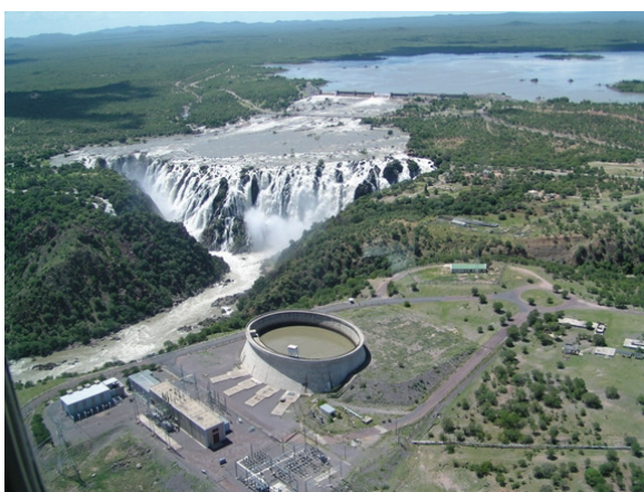
Figure 9: Ruacana Power Station in the North West of Namibia. A hydro energy source.
