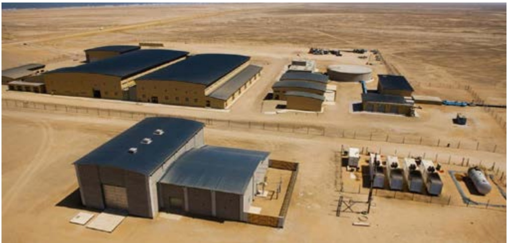
Figure 133: The Erongo Desalination Plant [Source: Orano]
