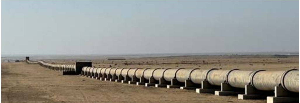
Figure 135: Connecting the water source with the distribution centre [Source: D von Oertzen]
