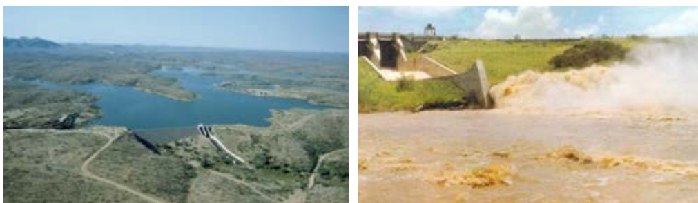
Figure 37: Von Bach Dam (left), and the Von Bach Dam spilling (right) [Source: DWA]
