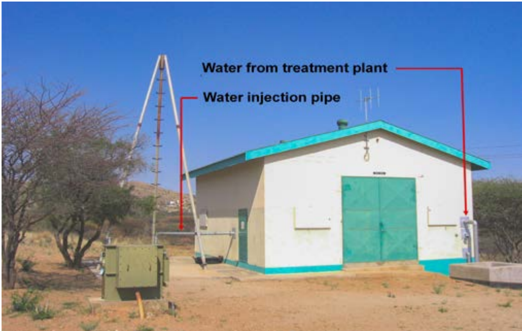
Figure 14: Artificial aquifer recharge station [Source: P Heyns]
