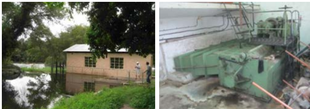
Figure 50: Andara power station, Okavango River (left) with 50kW generator [Source: P Heyns]
