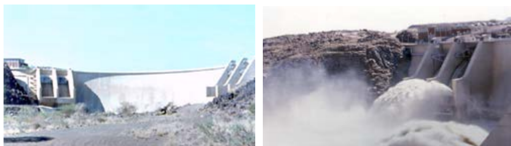
Figure 40: Naute Dam (left), dam spilling (right) [Source: P Heyns]
