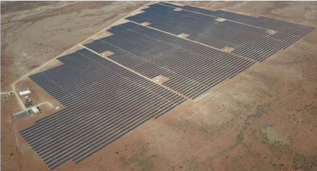
Figure 74: The 37 MW Alten solar PV plant east of Mariental [Source: C Roedern]
